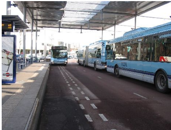
TEOR on the two-way reserved lanes, common section, Mont Riboudet station Source Certu
